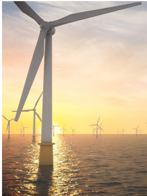
(Photo: Artistic illustration of wind turbines and a substation at Dogger Bank Wind Farm by Aibel)
